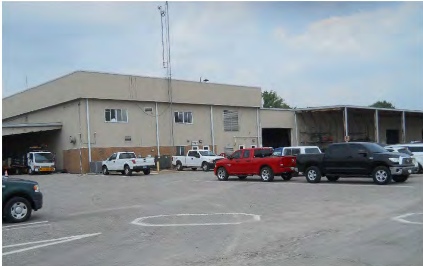
City garage – view looking northeast of the two-story office
