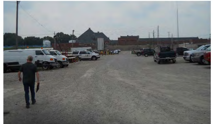
View west with the water treatment plant in the background
