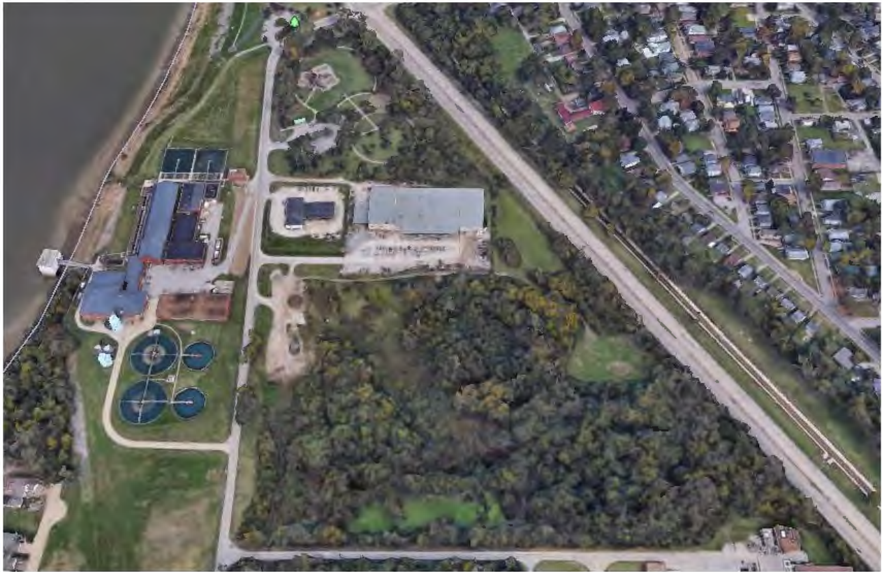
Pre 2019 aerial view
