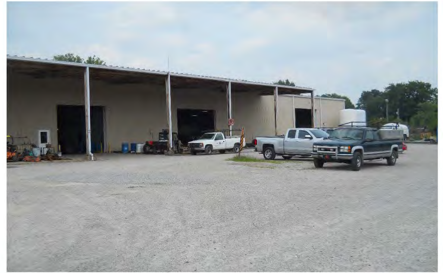
City garage – view looking northeast of the south canopy
