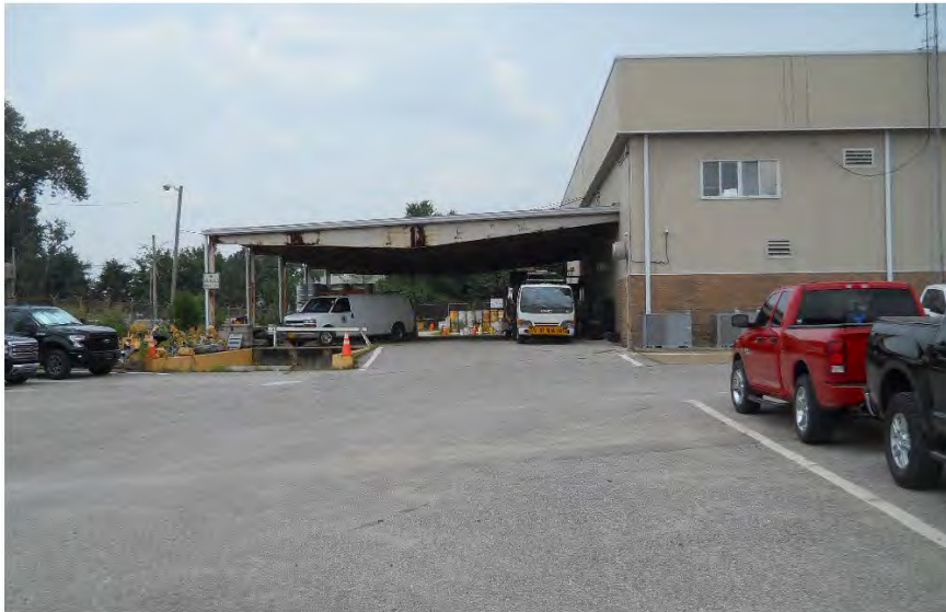
City garage – view looking north (OUCC photos - July 21, 2021)
