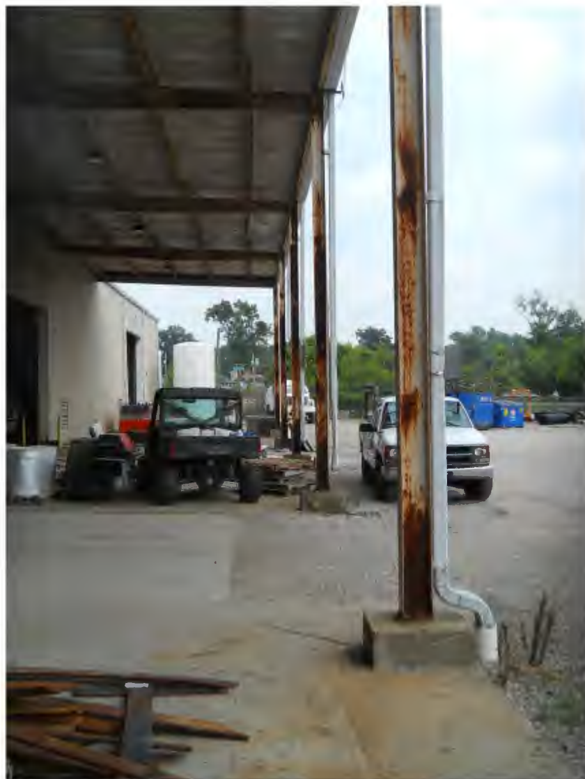
City garage – view looking east
