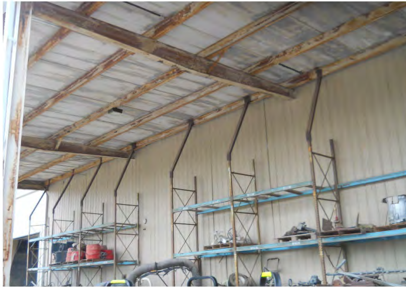
City garage – view showing the condition of the south canopy
